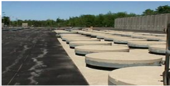
Higher-activity, longer-lived radioactive waste stored in in-ground containers
